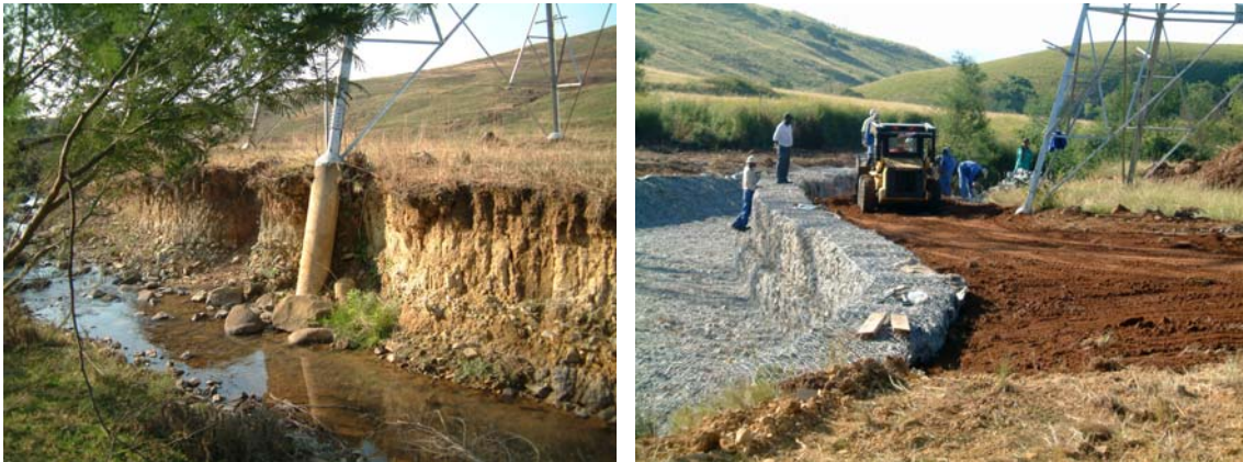
Figure 1: The photo on the left shows the foundation of a tower exposed by erosion. The photo on the right shows the extensive and costly remediation by using gabions and reno mattresses. Also note the use of good topsoil that will permit the re-establishment of vegetation around the tower (photos Jorge Correia).
