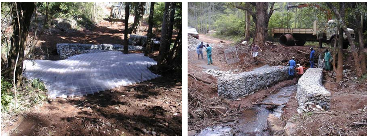
Figure 3. Extensive measures taken to prevent erosion, during the construction of access roads for a new power line. Continuous cellular mat (left) and gabions (right) are some of the measures used during the building of access roads during the construction phase of a power line. (Photos: Jose Clara).
