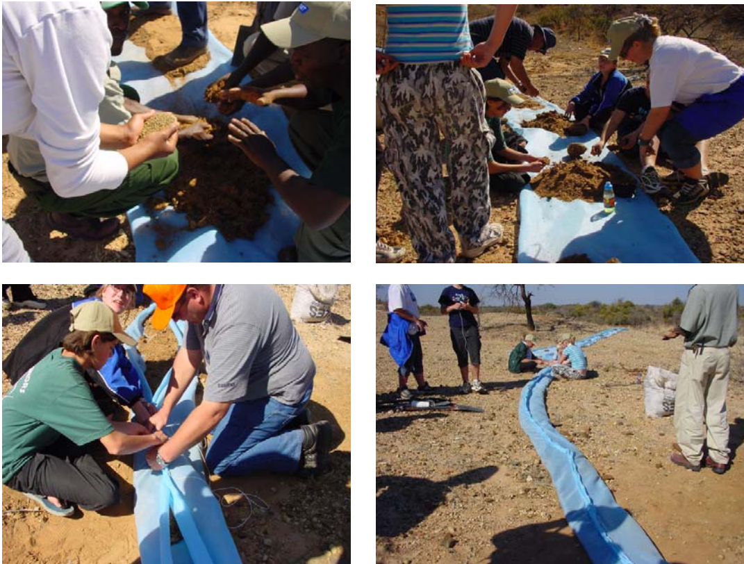
Figure 8. The photo's show the mixing of the soil, the manure seed and silicate mineral before placing it in the geotextile bags.
