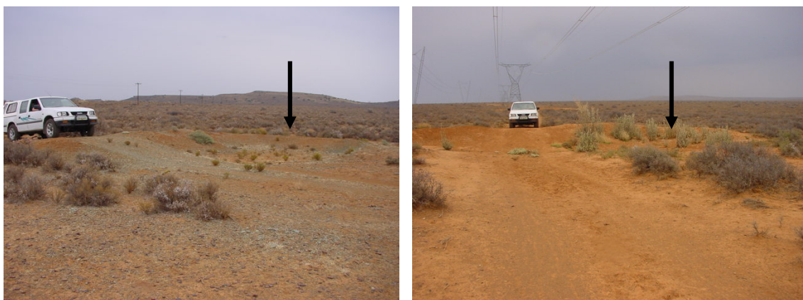
Figure 4. Examples of well constructed berms under the Hydra-Droërivier 1&3 lines. This design uses an overflow dam to spread water collected by the berm (see arrows). After ten years virtually no maintenance is required on these structures.
