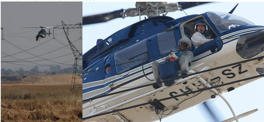
**Figure 2222: The installation of flappers on the shield wire from a helicopter.**
