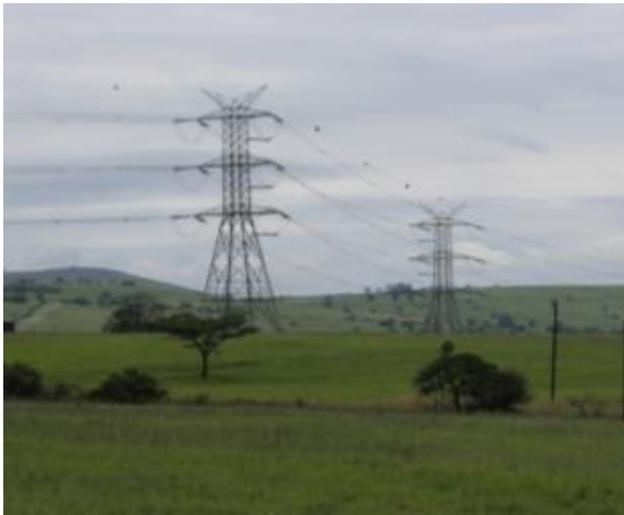
**Plate 6 Double-circuit 400 kV transmission line**
