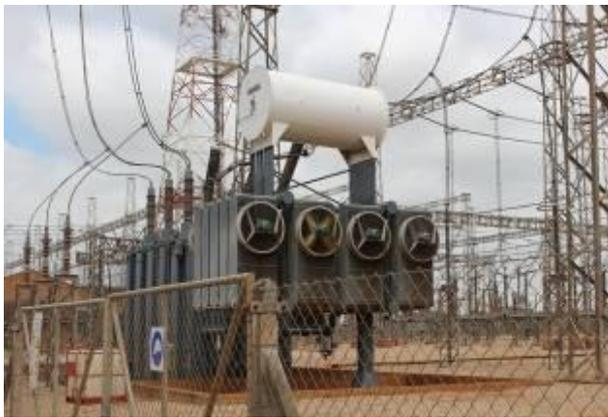
**Plate 3 Transformer showing oil storage and fans for cooling**
